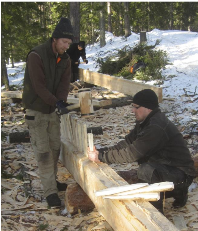
Figs. 17–18. Use of wedges and spårning . After initial spårning , a lot of wedges were used to get an even pressure. After a while we could concentrate more on spårning and used fewer wedges. The wedges we used were made of aspen. A good width of the wedges is two to three inches and thickness around one and a half inches, and the length approximately twelve inches. Photos Karl-Magnus Melin.
