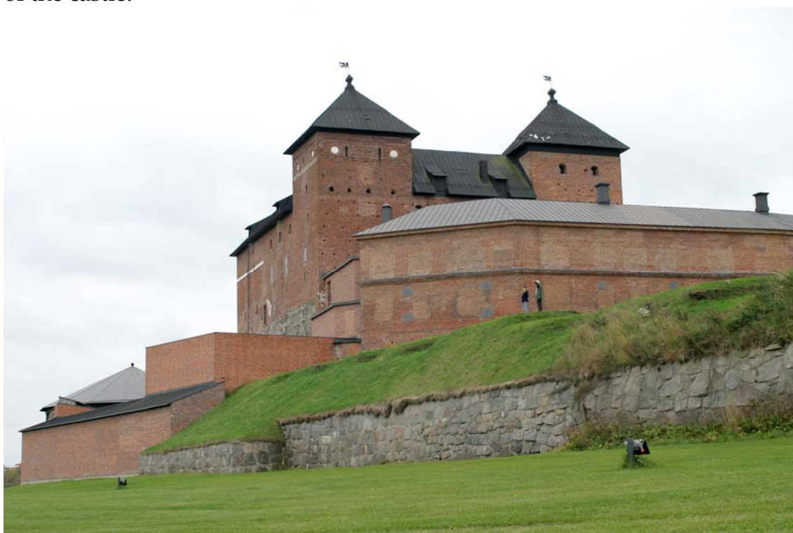
Picture 3. Häme Castle from the north. The ramparts in the foreground were built in the eighteenth century, as was the brick building in front of the castle. Photograph: Martti Lampila (NBA, Häme Castle).
