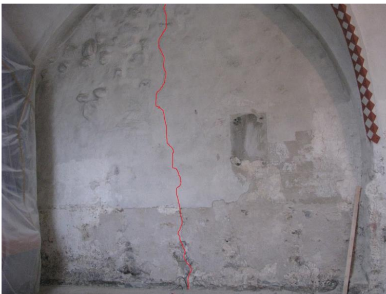
Fig. 17. Snesere church. The crack in the north wall of the west end of the present nave. Photo Nationalmuseet 2013.
