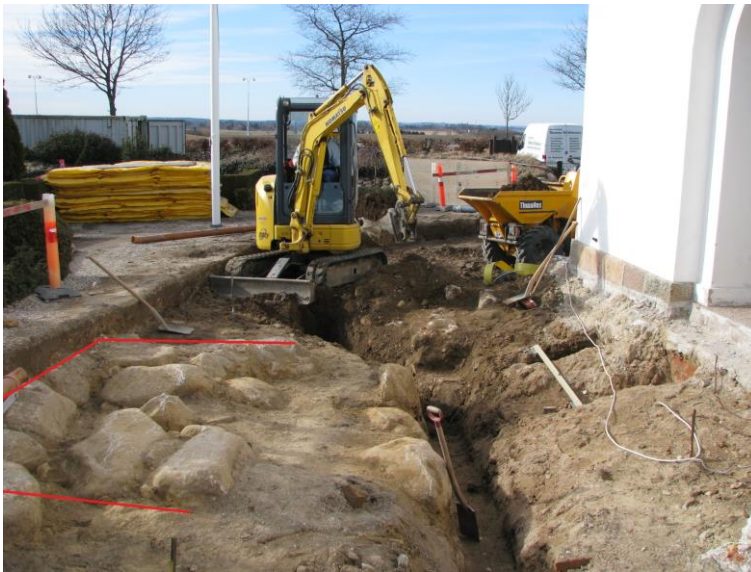
Fig. 6. Kirke Hyllinge church, south side of the present tower, seen from the east. The red line indicates traces of mortar. The entrance door is situated in the present tower. Photo Nationalmuseet 2011.
